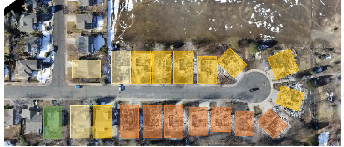
Proximity of homes to other damaged homes
