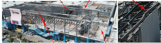
Total Loss of Purlins in Bay Buckled Diaphragm Collector
