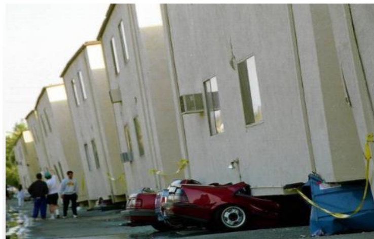
http://seblog.strongtie.com/tag/northridge-earthquake/ A row of buildings after the Northridge 1994 earthquake
