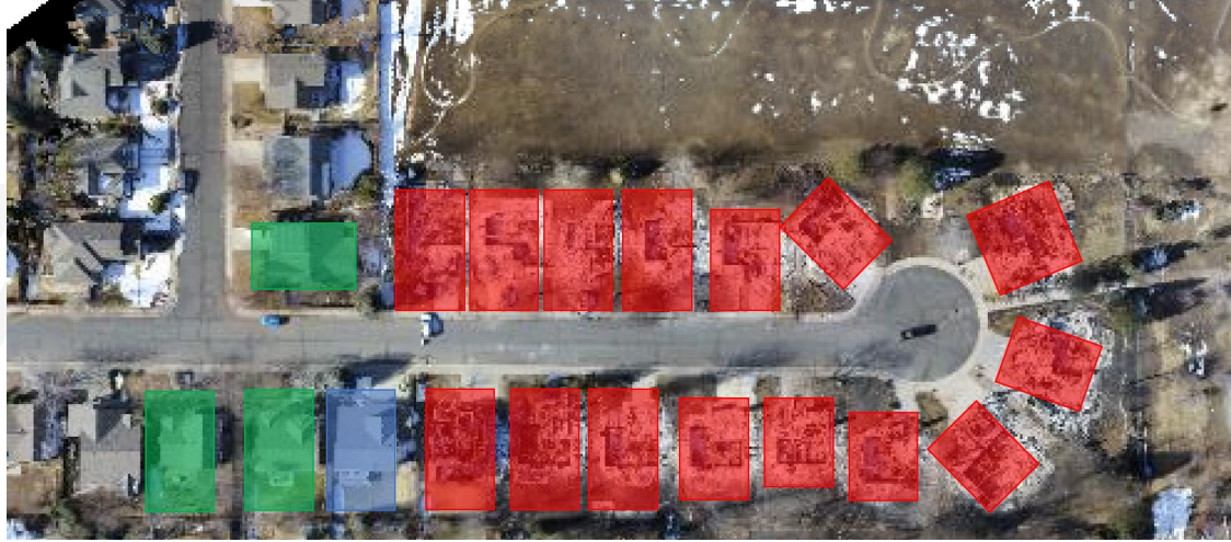
Damage state of homes
